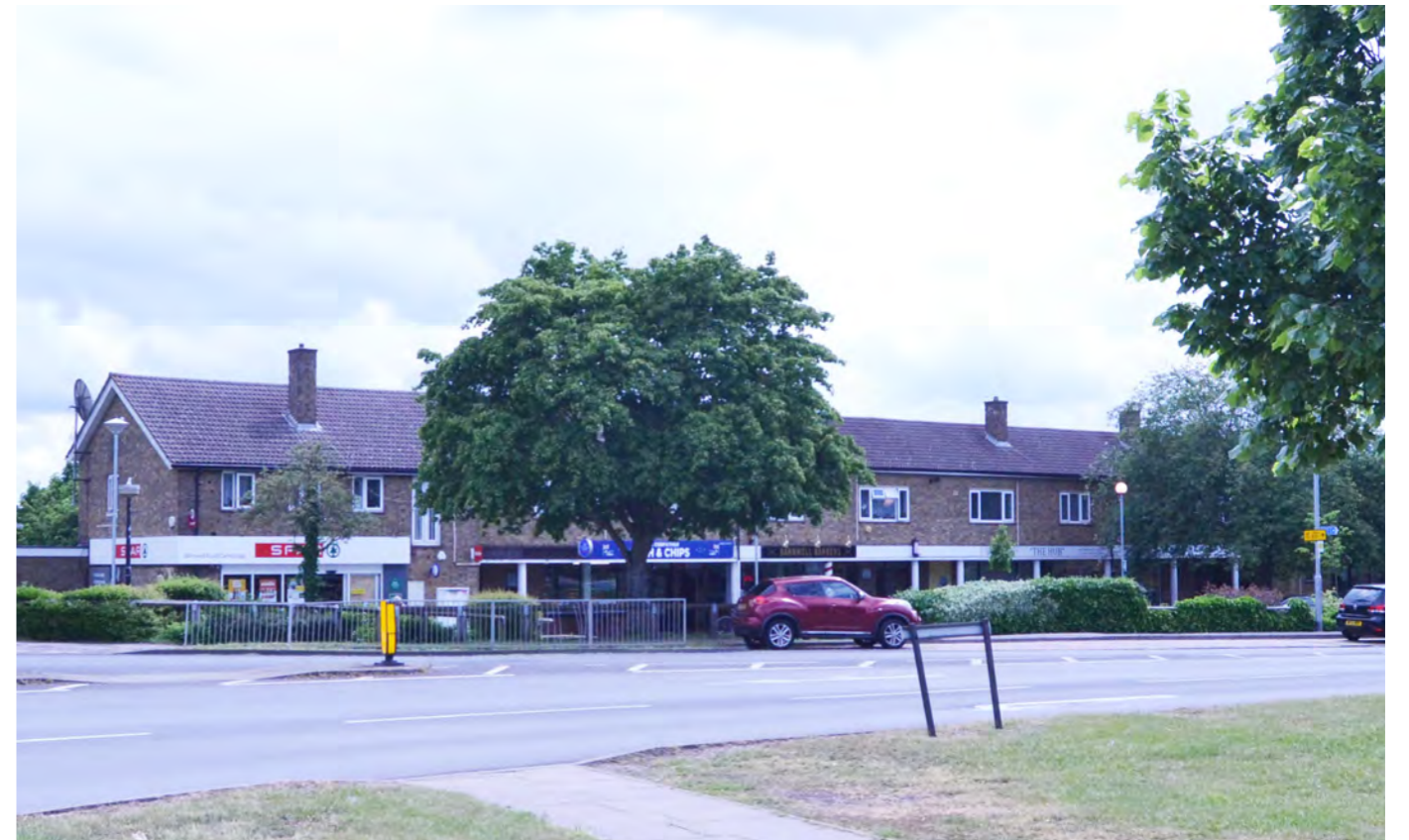
Site 2 - View of existing shops
